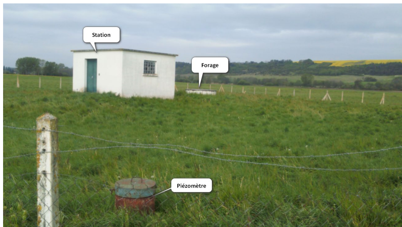
Figure 11 : station de captage.
